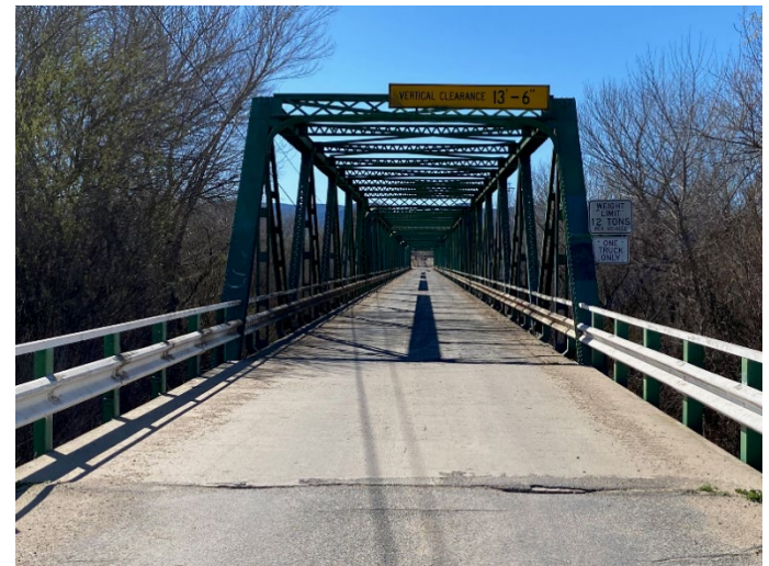
Facing San Lucas Bridge
