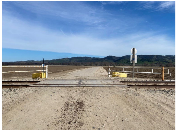
Access Gate to River
