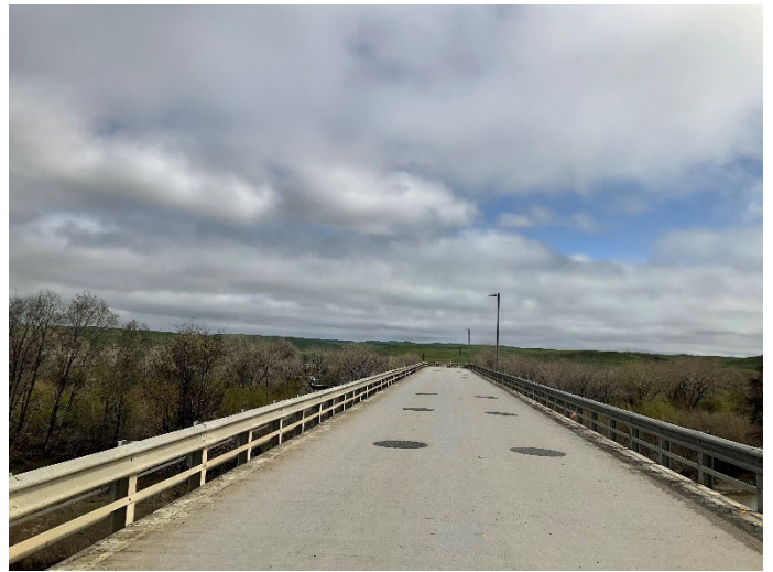
Bridge facing Oil Field
